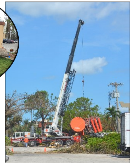
Telephone tower on ground; temporary smaller tower erected
