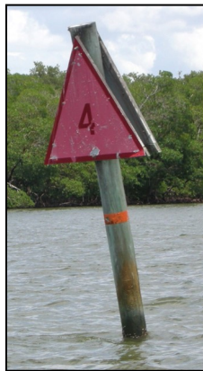
Temp Coon Key Light with submerged hazard; Leaning ATON “4” (reported; co-op charting)
