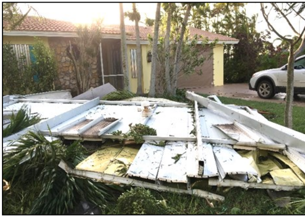
Gloodt's lanai and roof landed in front yard!
