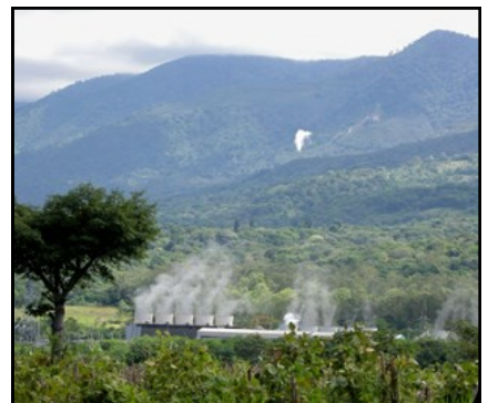
Geothermal plant; steam vent
